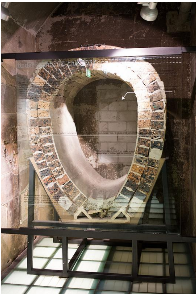
Figure 2.8: Section of brick oviform drain from arched stone section of Tank Stream. Google
