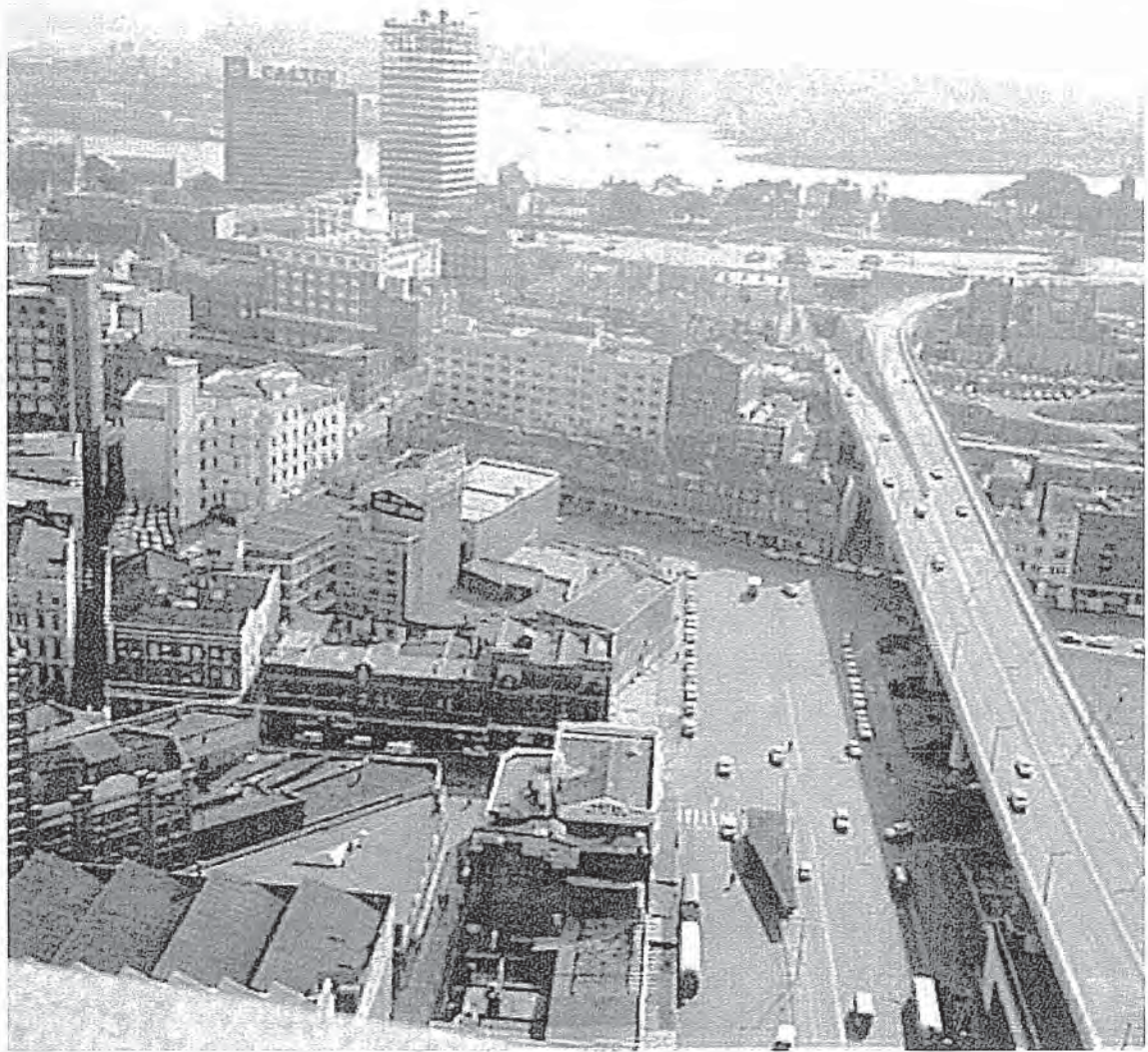
Figure 3.14: Aerial view west along Alfred Street, showing the site on the corner of Alfred, Pitt and George Streets. The completed Cahill Expressway is on the right. (Source: City of Sydney Council Archives)
