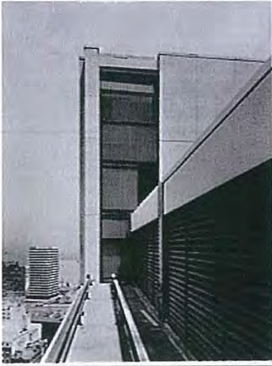
Figure 6.10 The modernist city, the air conditioning louvers on Gold Fields House demonstrating the new, sleek skyscraper design. (Source: City of Sydney Archives)
