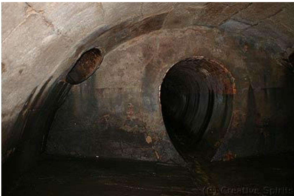
Figure 2.8: Section of brick oviform drain from arched stone section of Tank Stream. Google
